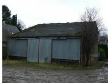
Above - Former barn materials
